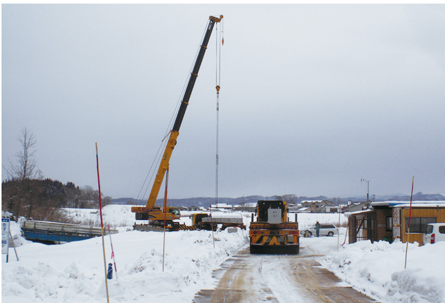
橋梁本体設置
